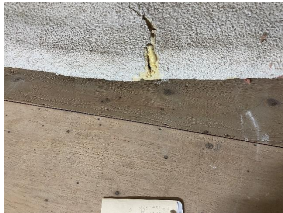
Foundation footing on east side is pushed inward and broken.
