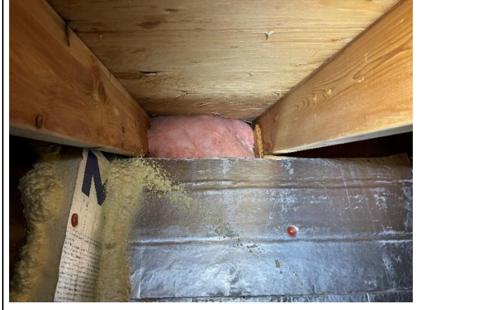
Rafter space over loft. Hot roof.
