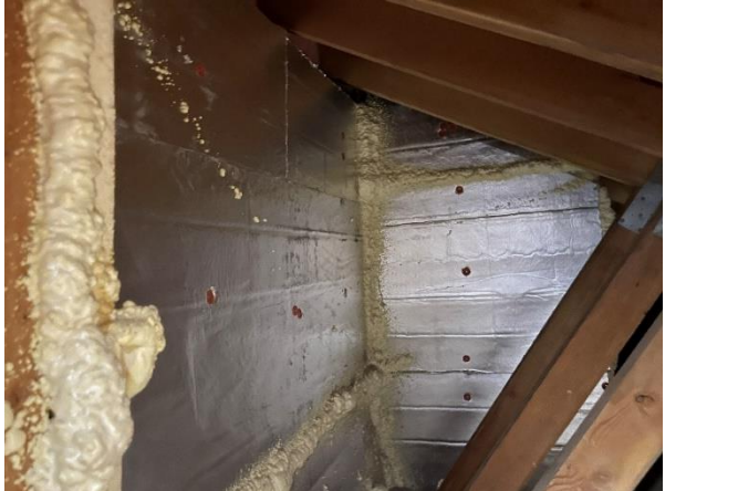
2" of polyisocyanurate insulation on loft walls
