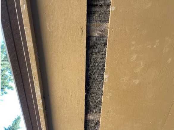
Clean the soffit vent screens
