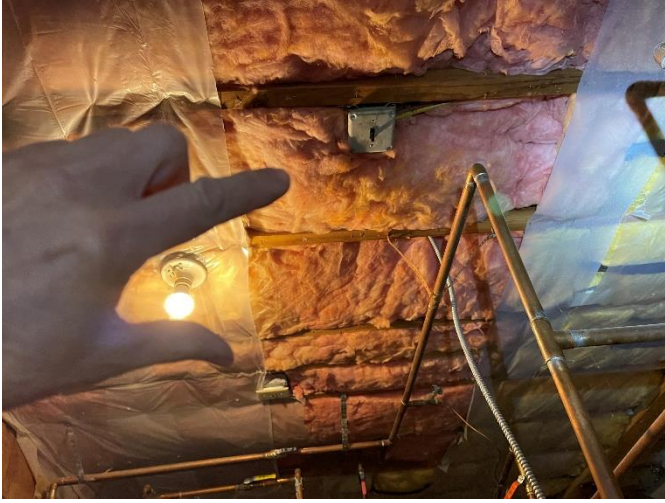
Label switches in the ceiling of the crawlspace.
