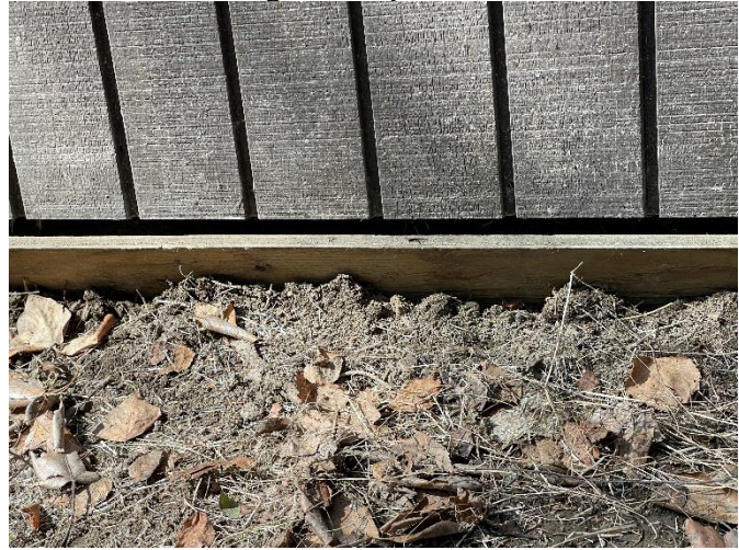
Top of foundation wall pushed in on the east side. The bottom footing is also pushed inward.
